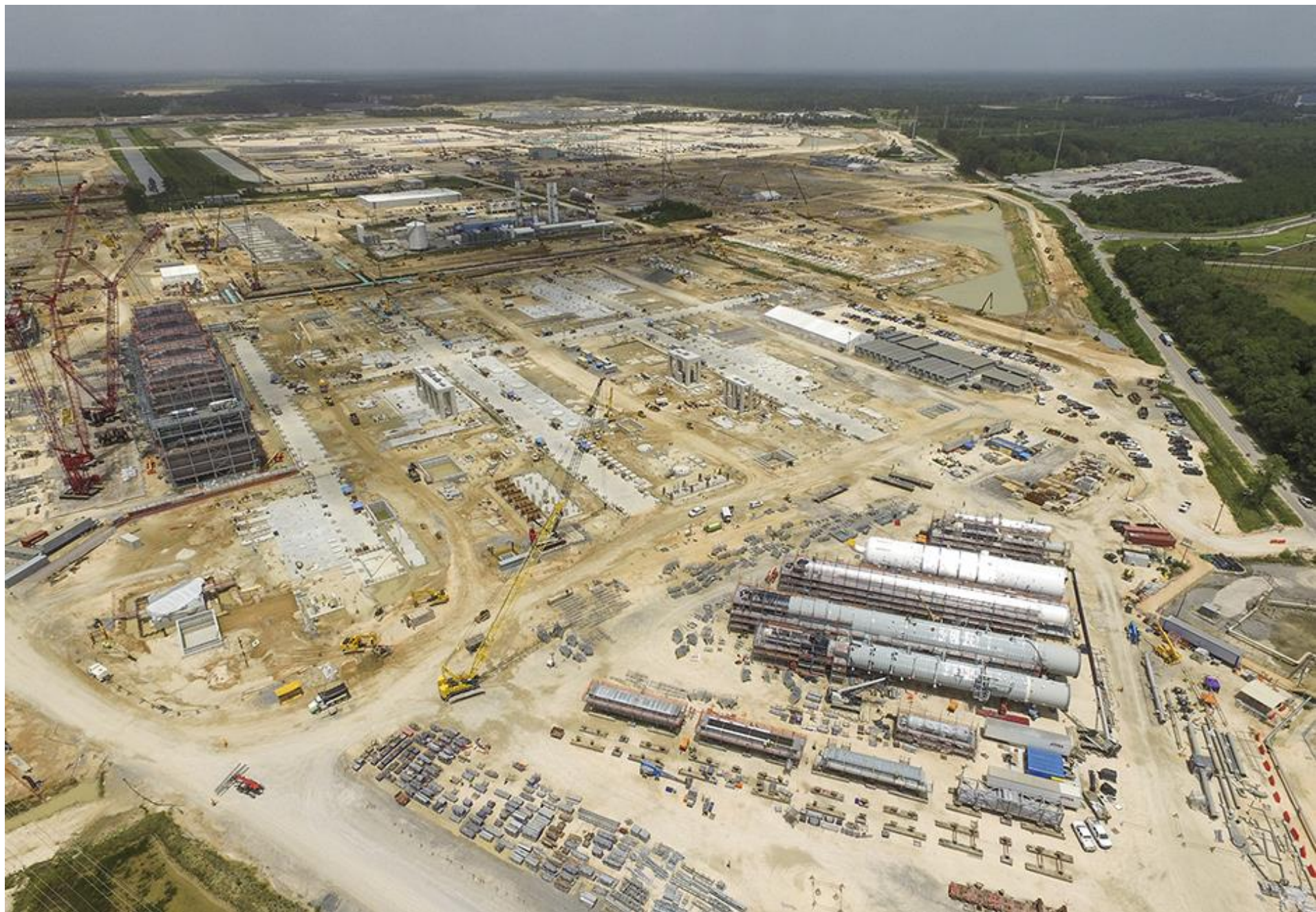
Project site, LCCP, USA
