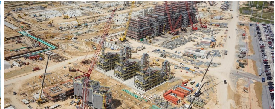
Lake Charles Chemicals Project, Lake Charles, USA
