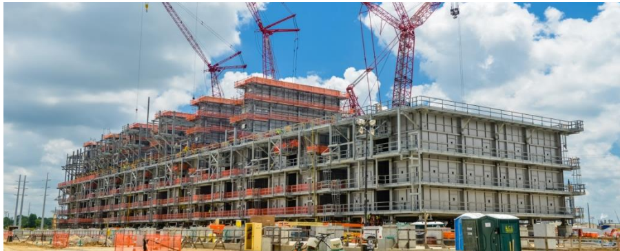
Lake Charles Chemicals Project, Lake Charles, USA
